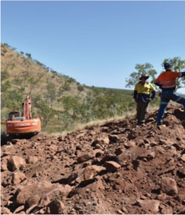
Re-contouring of a cut and fill exploration drill pad
