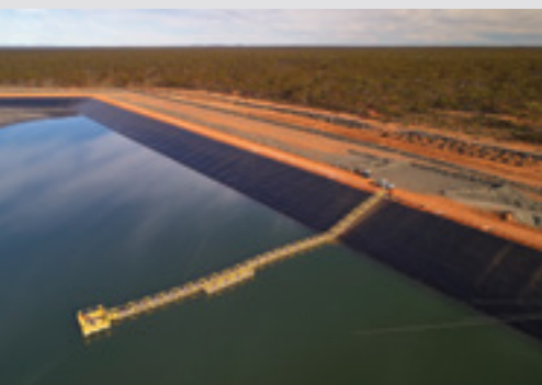
Nova Operation Tailings Storage Facility
