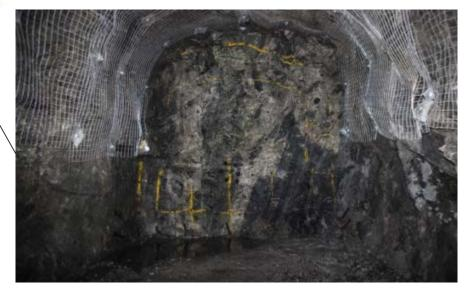
28 June 2016: Brecciated Sulphide in Sed-Sed contact
