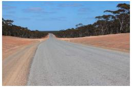
Sealing works on the Project's 38km access road through to the Eyre Highway is currently underway and is expected to be completed by early December. Work on rehabilitation of temporary construction areas established for the road's construction has also commenced and is planned to be completed by the end of the year.
